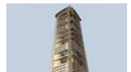
AbbcO Tower at Al Nahda Sharjah
