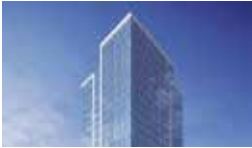
Al Huwailah Towers at Al Mirqab Qatar
